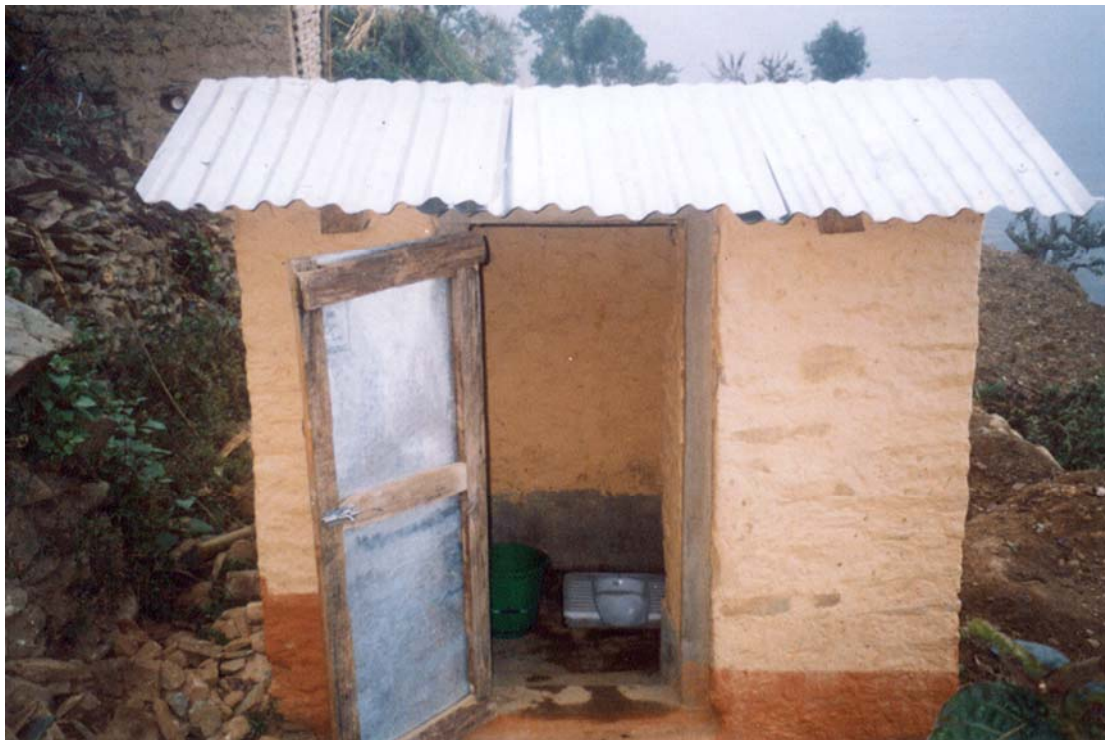
COMPLETED TOILET BUILDING
