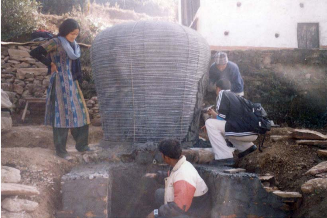
RAINWATER HARVESTING STORAGE TANK UNDER CONSTRUCTION
