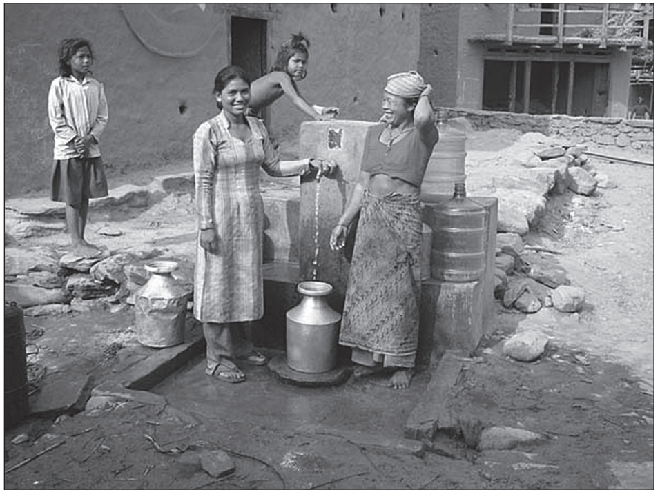
The people of Kunauri still make good use of the water system installed 18 years ago. The current World Neighbours Canada project in Nepal has expanded beyond water systems and now includes providing the pipe and water trap for simple latrine systems. All the families in Kunauri have now installed latrines.
