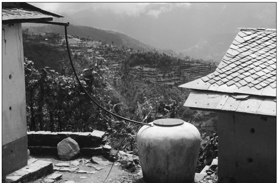
In those villages without access to gravity fed water sources, the alternative is to construct rain water harvesting systems. Rain captured from the roof is fed into a simple ferro-concrete tank. The current three-year project with CIDA assistance is implementing both water systems and latrines.
